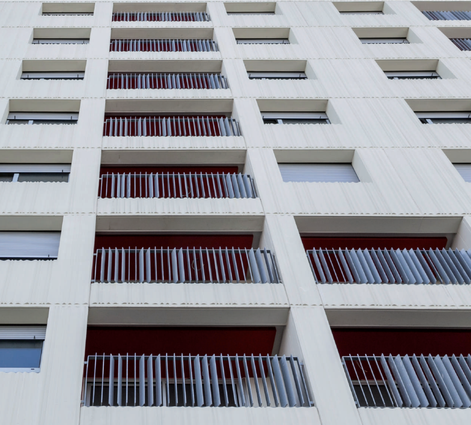
Facade of the Ca l'Isidret public housing building, on the corner of Carrer Pere IV and Carrer Josep Pla.
