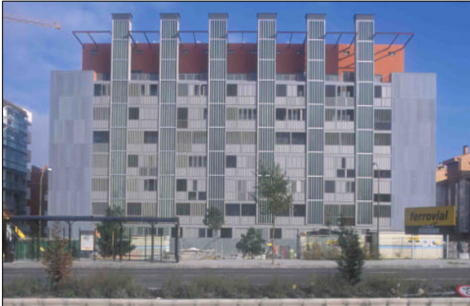
West facade of social housing project with solar exhaust chimneys
