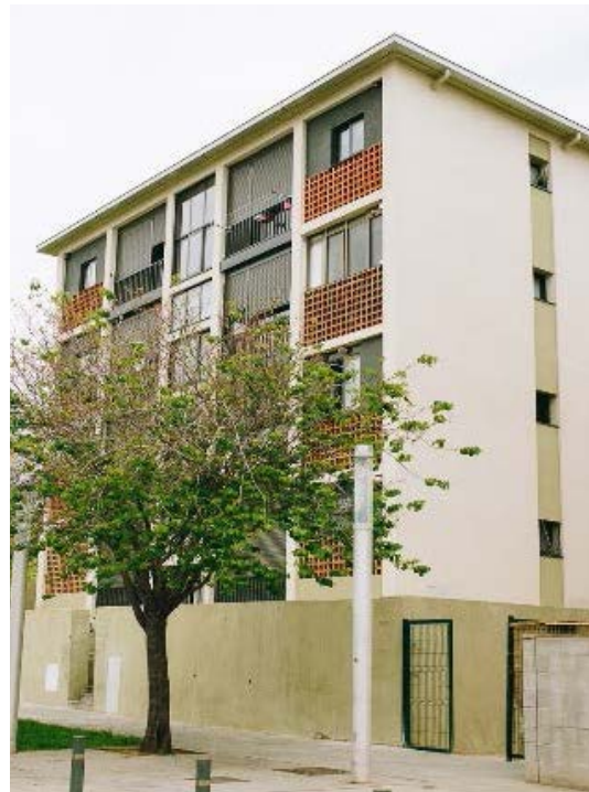
Fortuna renovation, La Marina
