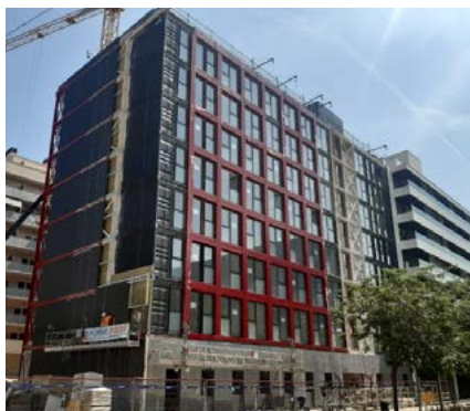
APROP in Glòries, under construction
