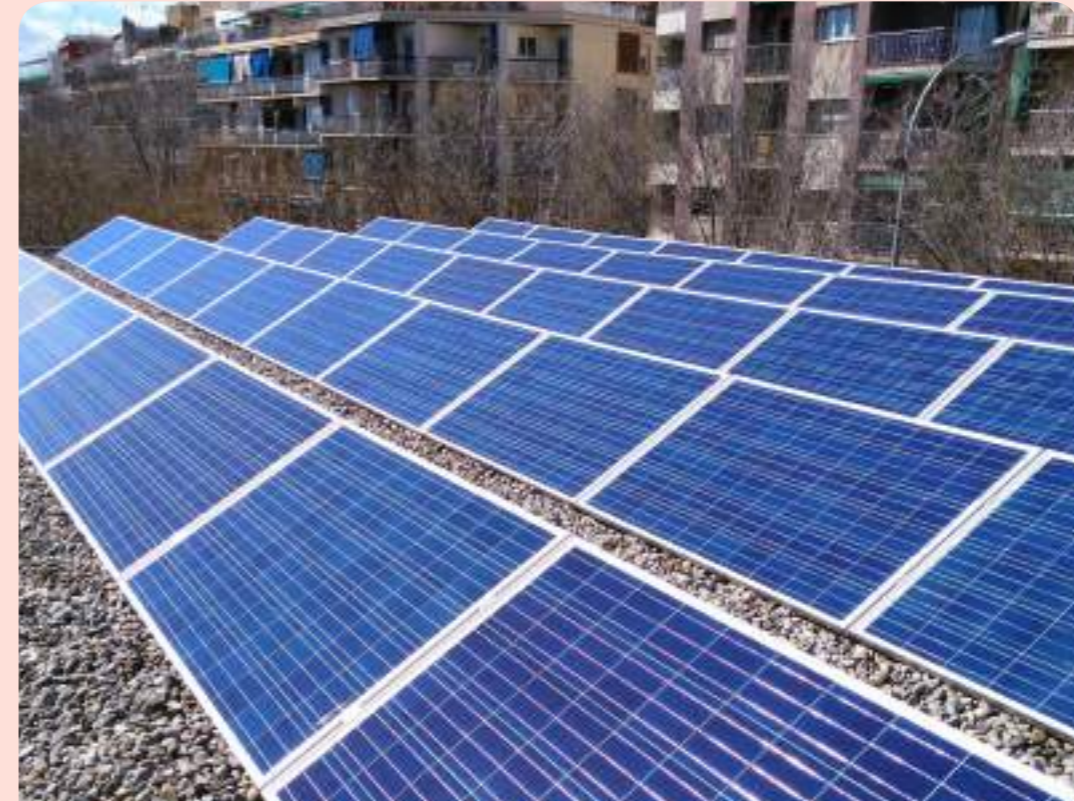
Improving energy efficiency
